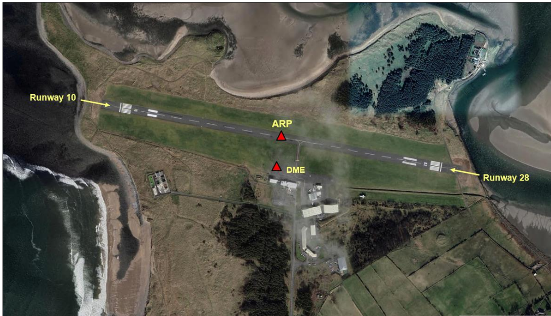
Figure 2. Sligo Airport - Aerial View
